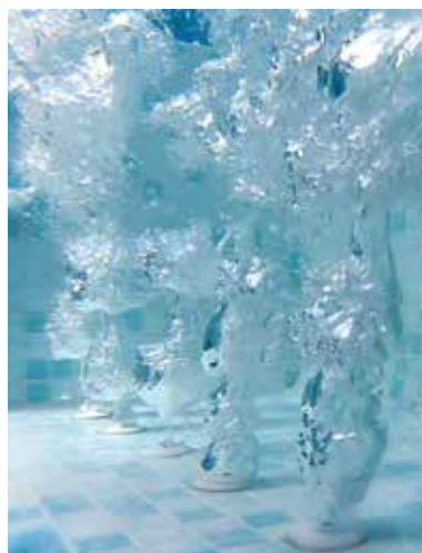
Closely spaced nozzles for an even spread of bubbles on water's surface
